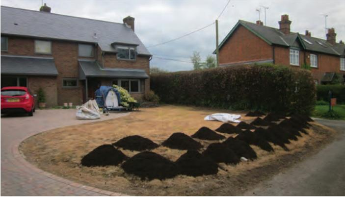
Fig. 12 Site 3 prepared by spraying and raking. (No rotavation.) Wildflower Earth product laid in April.
