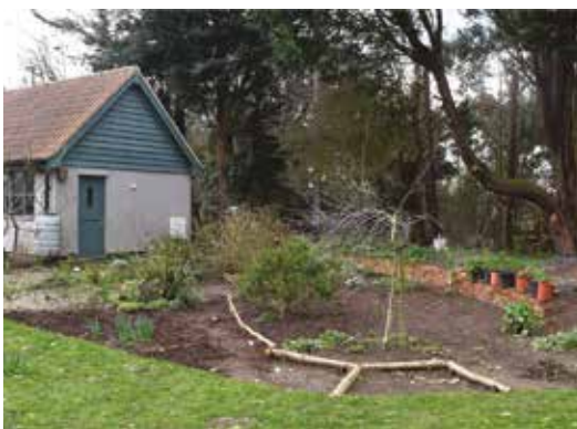
Fig. 18 Laying out the first gravel garden, March 2017
